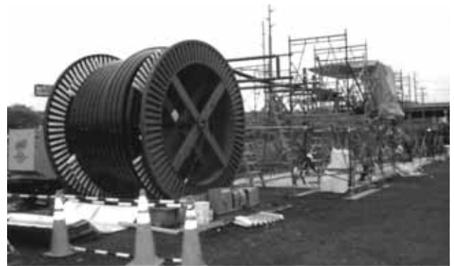
Photo 2. HTS Cable Installation
