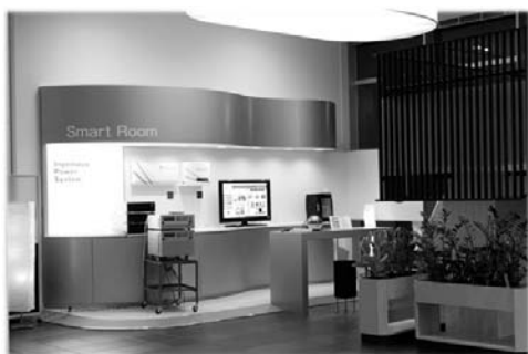
Photo 3. Inverter and loads
