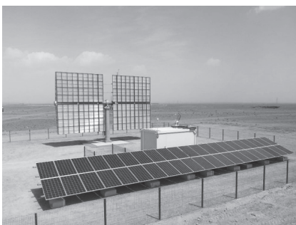
Photo 2. System installed in Ouarzazate (Back: 20 kW-class CPV; Front: fixed 10 kW Si-PV)
