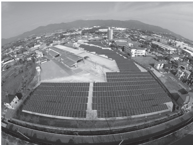
Photo 2. Overview of a 1 MW solar power plant
