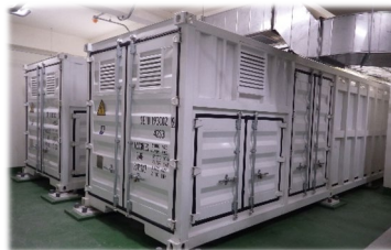
Shalun Smart Green Energy Science City in Taiwan
