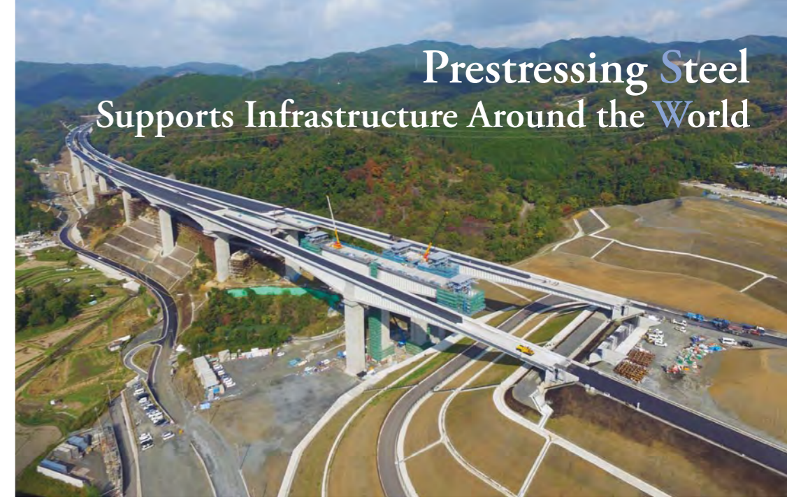
Youbaizan Viaduct (Photo courtesy of Sumitomo Mitsui Construction Co., Ltd.)
