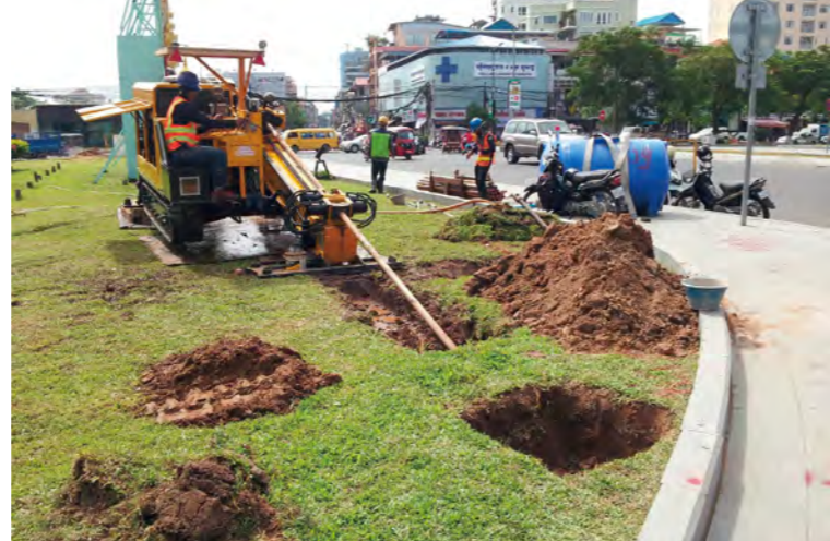
Horizontal drilling method enabled road work without disturbing traffic
