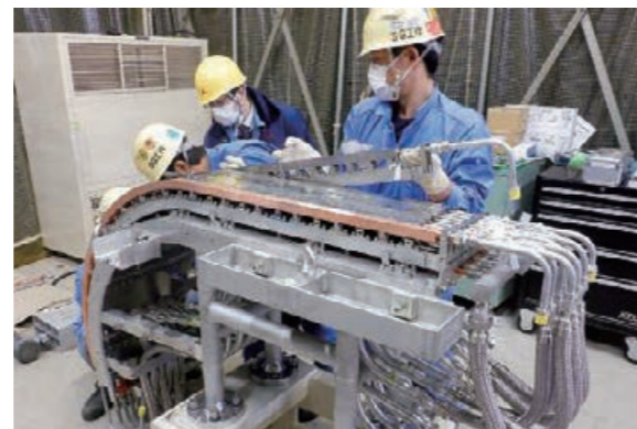
Installing monoblocks in the outer vertical target ©QST
