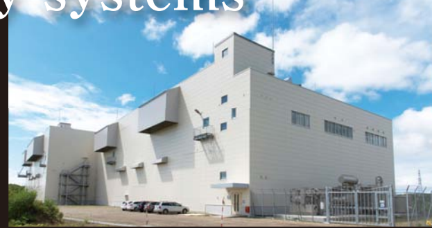
Building housing the storage battery system
