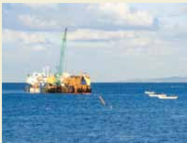
Submarine cable laying
