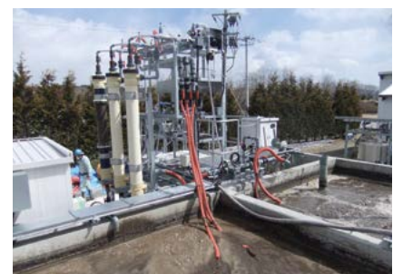
Simplified POREFLON™ MBR device that can be attached externally
