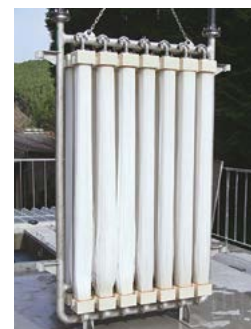
Water treatment membrane modules
