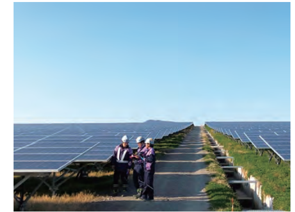
Construction work of a mega-solar system
