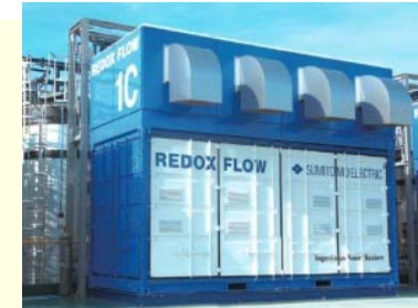
Redox flow battery
