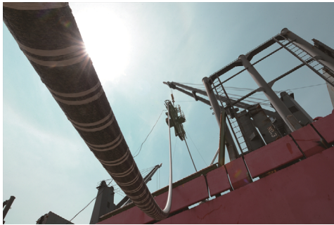
Photo 1. Submarine cable installation (NEMO project)
