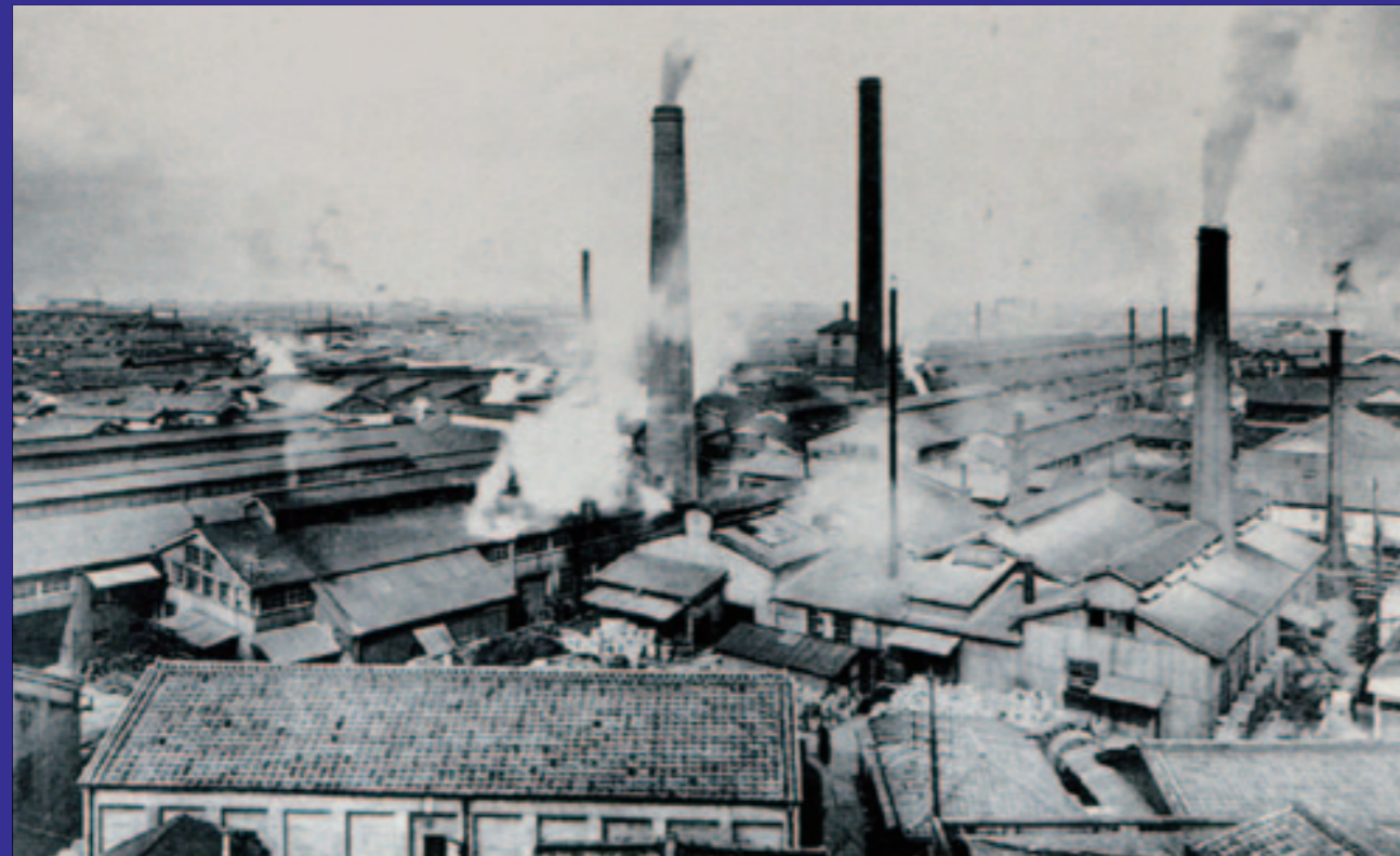
Full view of Sumitomo Copper Rolling Works in Ajigawa (Photo courtesy of Sumitomo Historical Archives)
