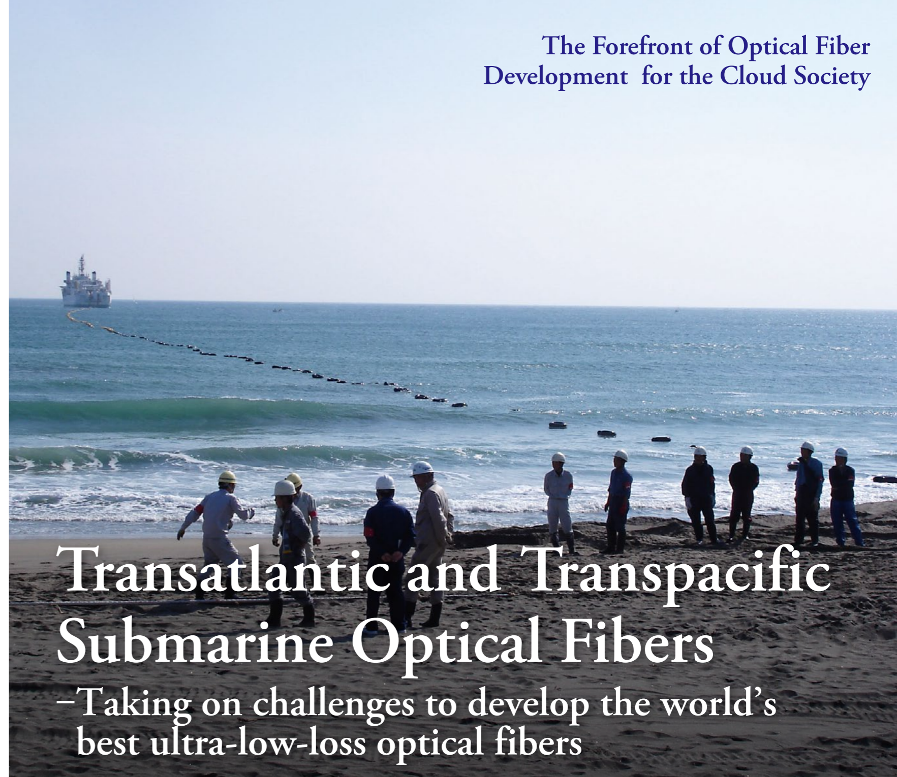
Submarine cable installation (photo courtesy: NEC Corporation)
