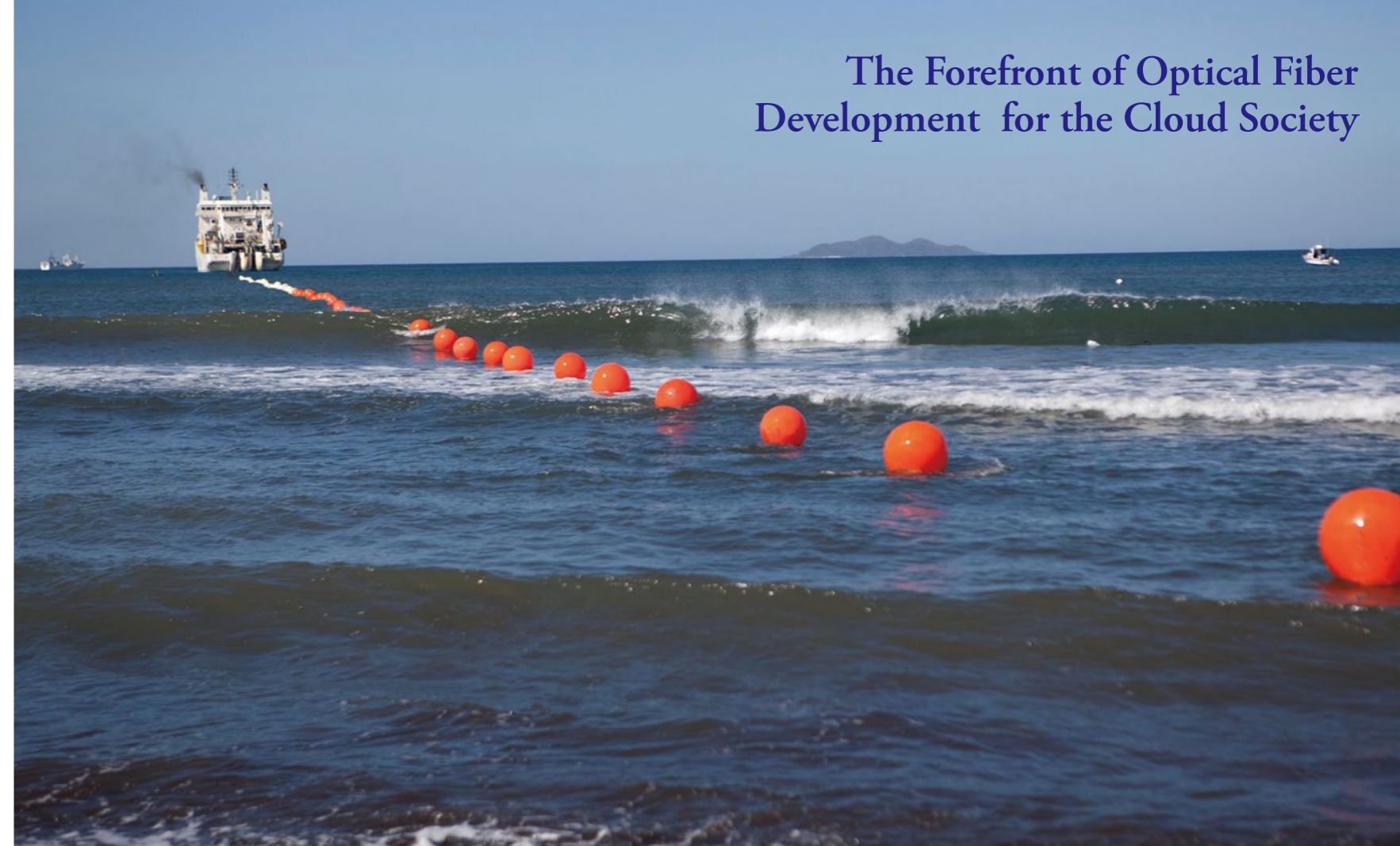
Laying a submarine cable (photo courtesy: NEC Corporation)
