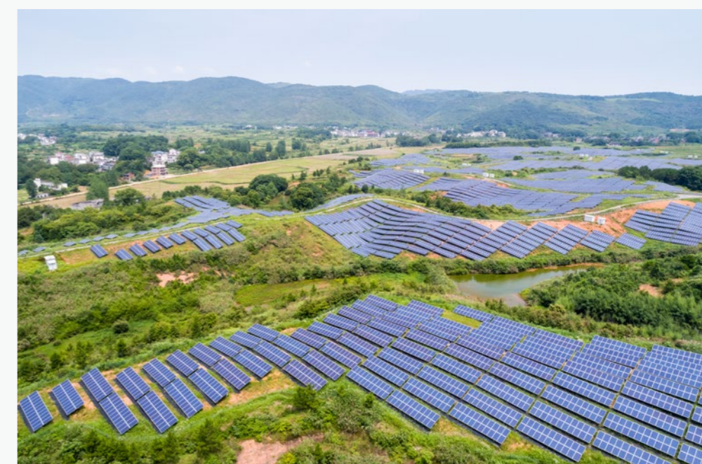
Abnormality detection is difficult in photovoltaic power plants where many photovoltaic panels installed in a large area are in operation.
