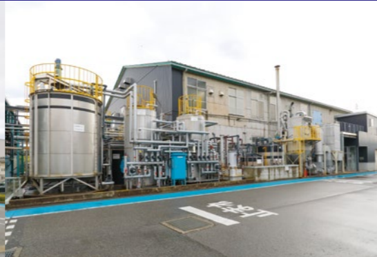
Overview of the new oxidation-wet chemical processing building
