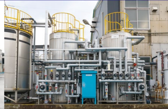
Ion exchange building
