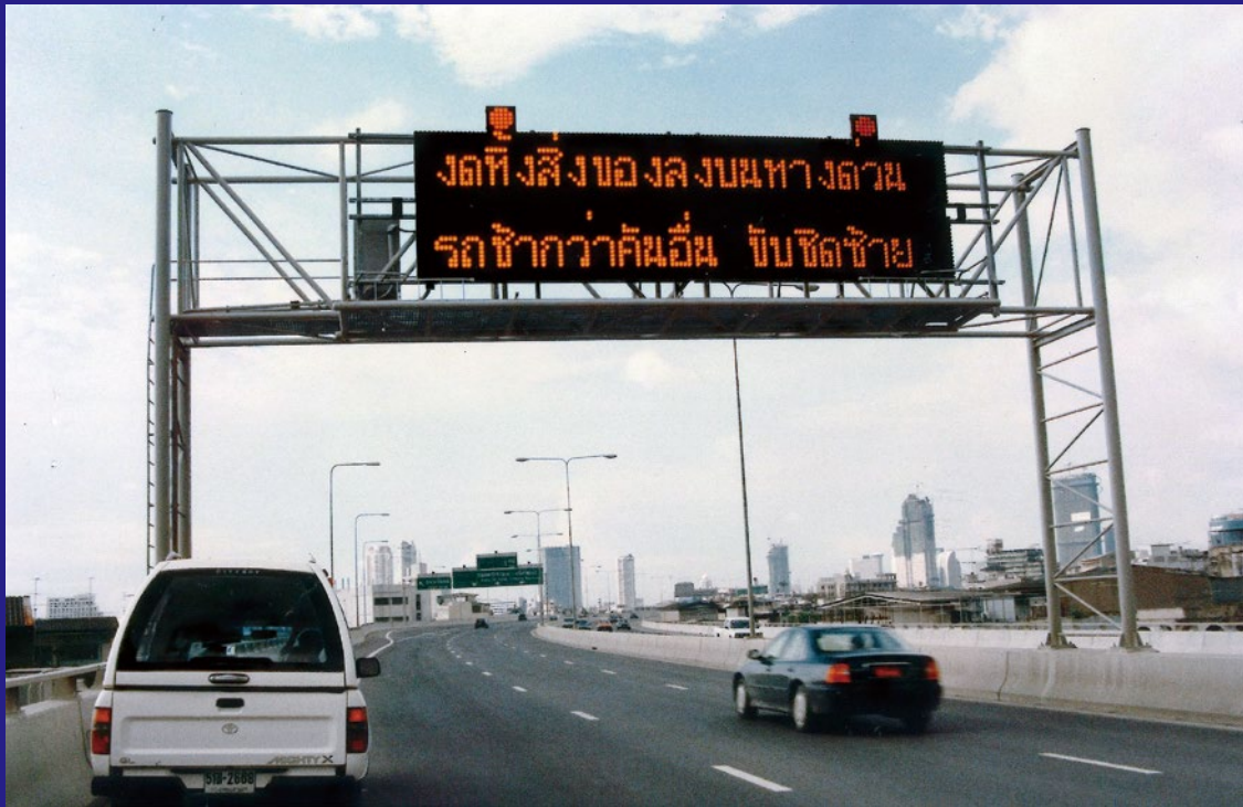
Multifunctional signboard of an expressway traffic control system
