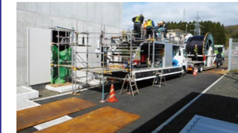
Installation (on the Hokkaido side: Yoshioka cable head (draw-in port))
