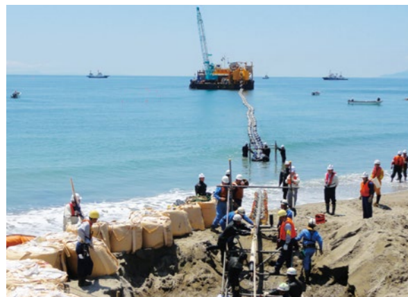
Cable installation for the Hokkaido-Honshu HDVC Link
