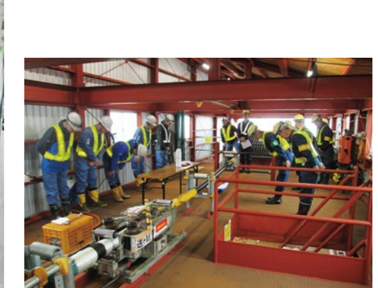
Ceremony to draw in the cable (Yoshioka construction base)
