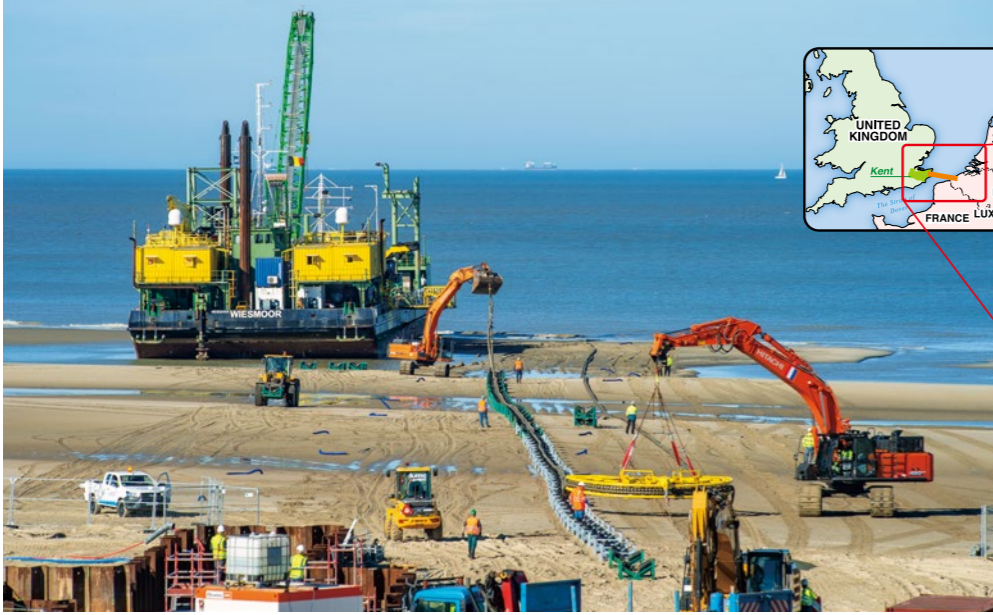
Cable laying on the Belgium beach side
