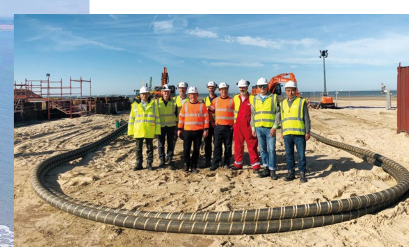
Construction proceeded with multinational members
