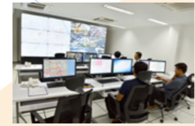
Traffic control systems These systems collect and analyze a wide range of transport information and use it to control traffic lights and provide transport information, enabling a safe and smooth flow of traffic.
