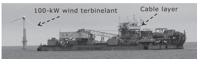
Photo 1. Cable laying to the 100-kW wind turbine
