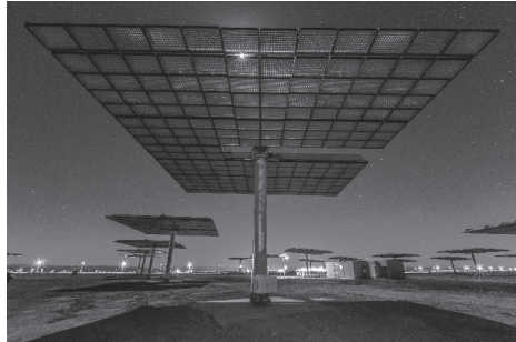
Photo 5. Night Stow Position with the Modules Faced Down
