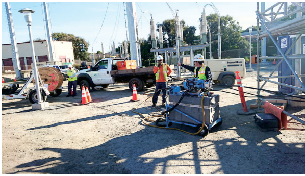
Photo 8. Installation of Optic cable
