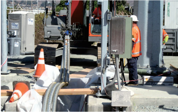
Photo 3. Removal of existing cable
