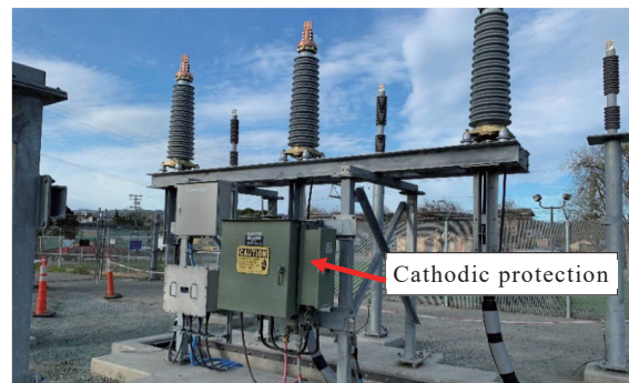
Photo 7. Assembled termination
