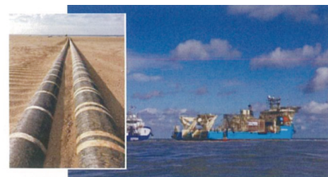
Photo 2. Cables laid in the shore section and a cable laying vessel
