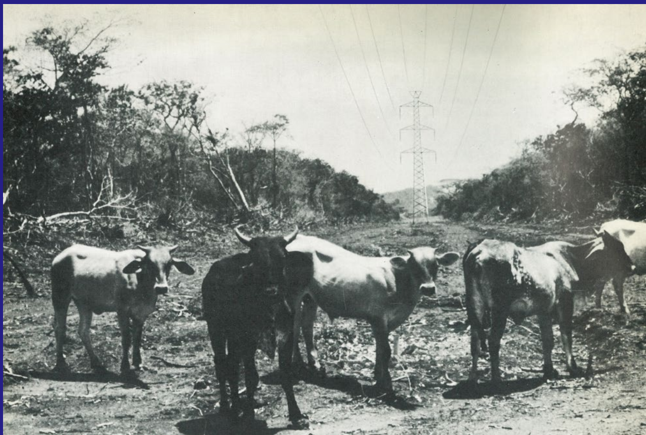
Conductors installed in Caroni, Venezuela
