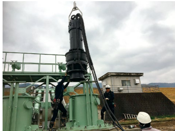
Installation of the pump and the inside of the pump. Highly accurate diameters of the S-FREE™ cables (black cables) ensure water sealing. (Photo and illustration courtesy of Tsurumi Manufacturing Co., Ltd.)
