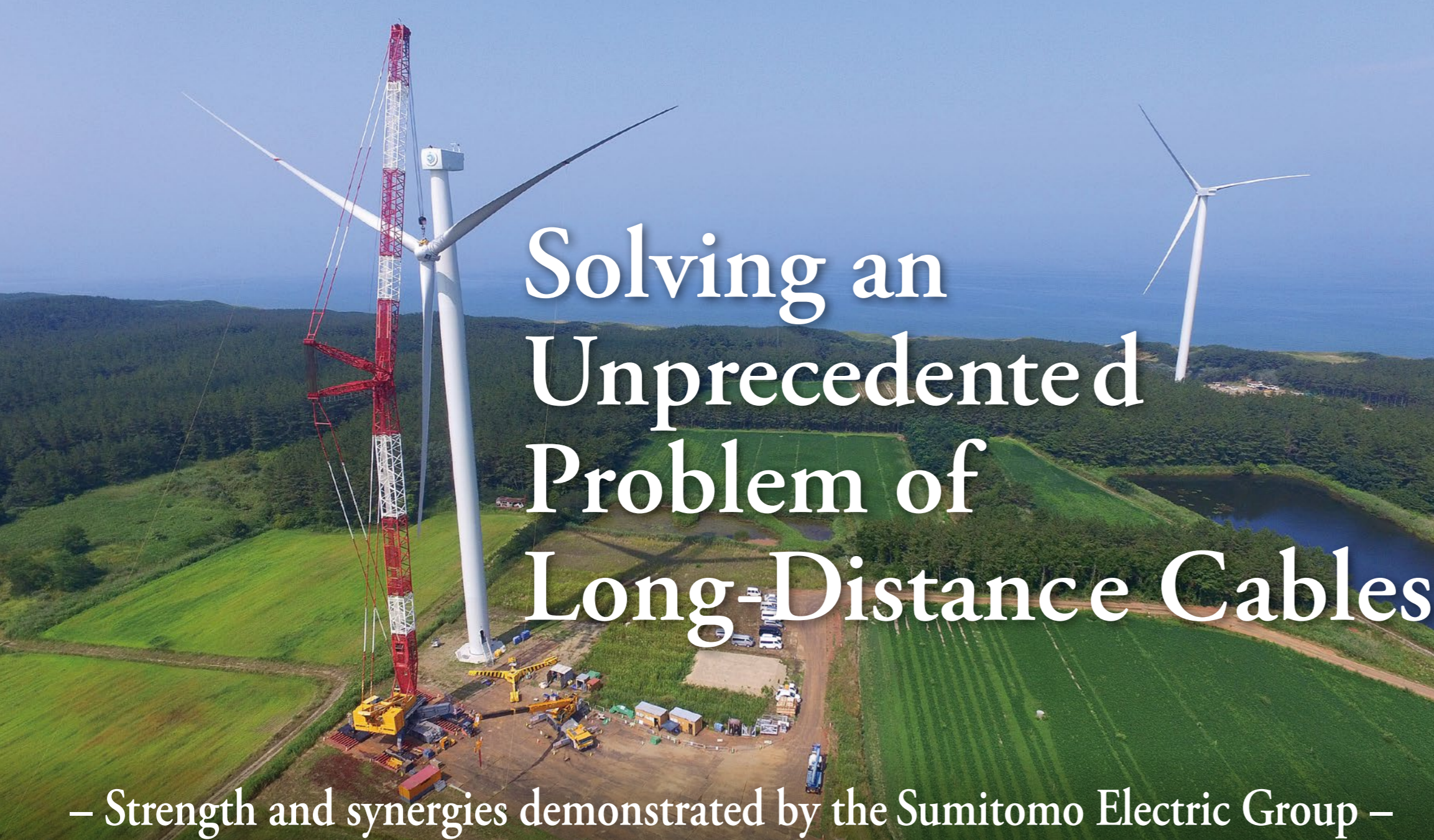
Wind turbine installation work(Photo courtesy of Kajima Corporation)
