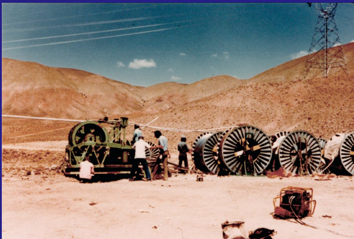
Construction of a transmission line completed under severe conditions in Iran
