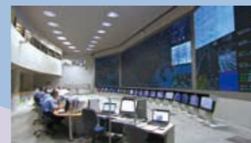
Traffic control system
