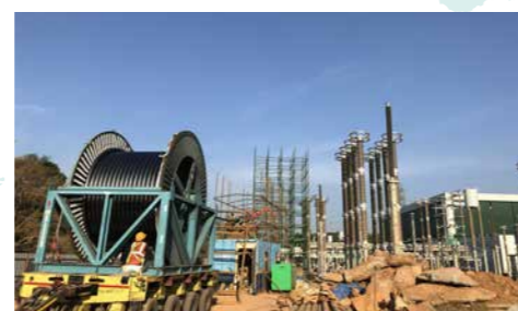
Cable installation site in India
