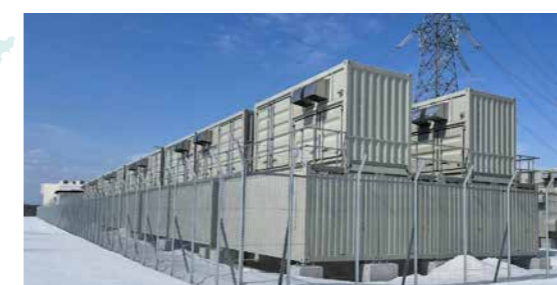
Redox flow battery system for Hokkaido Electric Power Network, Inc.
